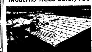
Boofers apply asphalt shingles to low-slope roof of new home.
