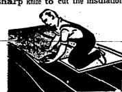
to the proper length and a piece of board to kneel on so you won't step on the ceiling. When the job is done, your mineral wool will start paying for itself in heat savings and will make your house more comfortable in all seasons. Mineral wool batts or blankets are recommended for open joists. However, if the attic has a finished floor, a professional installer can blow insulation into the hidden areas.
