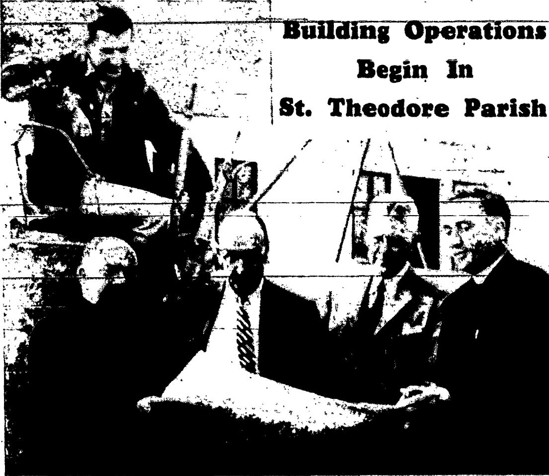
PLANNING GATES PARISH CONSTRUCTION — With work on proposed new church and school buildings for St. Theodore's parish scheduled to begin within a few days, priests of the parish are pictured conferring on the project. From left are the Rev. Raymond J. Epping, pastor; Carl Luther, of John Luther & Sons, contractors; Edward M. Lorscheider, architect, and the Rev. John J. Steggs, assistant pastor.
