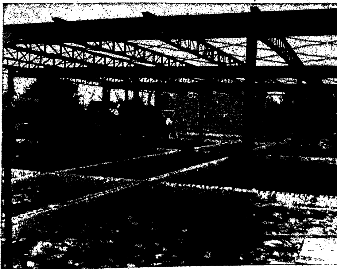
New School Rising In Irondequoit STEEL WORK for the auditorium of the new Christ the King Parish is being erected on 55th St. Highway, Irondequoit. Construction of the school is advancing and the church building awaiting delayed steel delivery. The Rt. Rev. Msgr. Charles J. Mahoney is pastor. (Paul Costantabile staff photo.)
