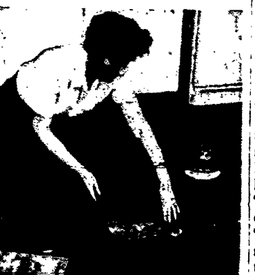
Setting the first tile
