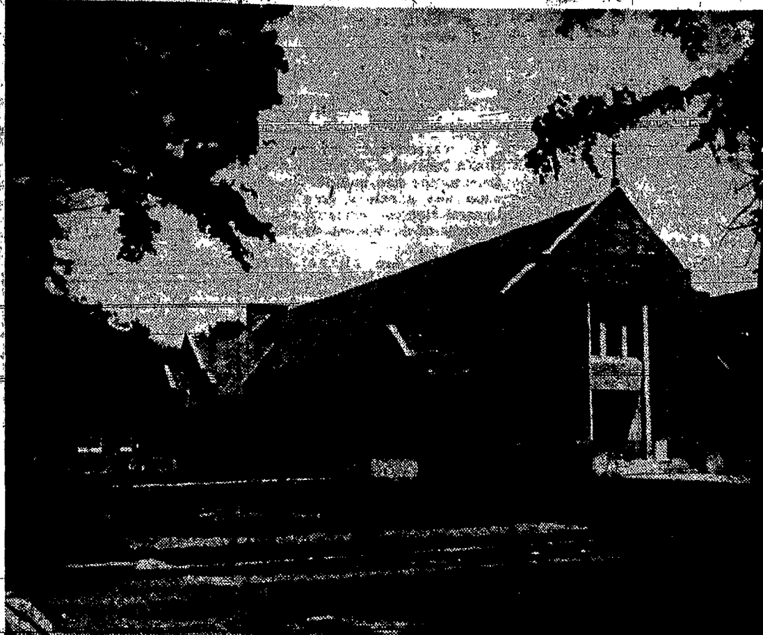
NEW CHURCH AND RECTORY for St. Vincent de Paul parish, Corning, will be blessed by His Excellency, Bishop James E. Kearney, Sunday, June 26, 11 a.m. Rectory is shown at left of picture above, at rear of new church. Rev. Joseph V. Guilfoil, pastor, directed design and construction of the $385,000 project. Old church will be converted into new classrooms for parish school use. (Faust Studio Photo)
