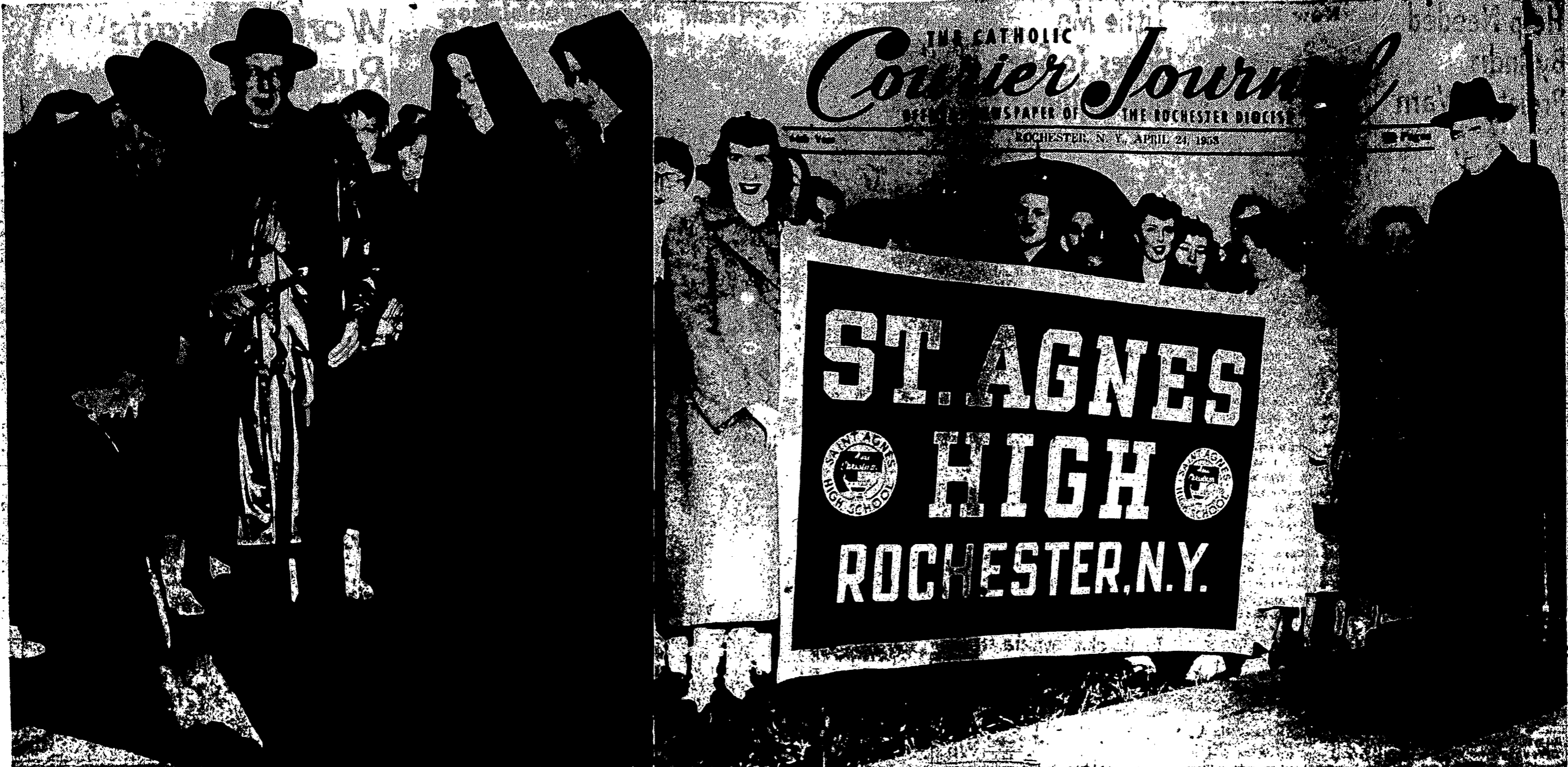
HIGH SCHOOL LAUNCHED — His Excellency Bishop Kearney (photo left) defied the rain to break ground Wednesday afternoon for the new St. Agnes High School
