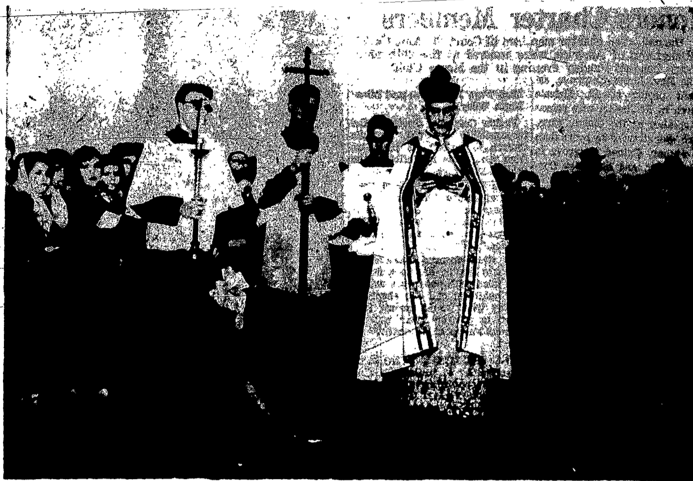
Site of the new Notre Dame de Lourdes High School on Lower Maple Ave., Elmira was blessed Feb. 11 in formal ground-breaking ceremonies. The Rt. Rev. Msgr. William J. Brien, V.F., dean of the Elmira Deanery and pastor of St. Patrick's Church, is shown offering a prayer as part of the gathering of 1,500 looks on. Immediately behind the Monsignor are, from
