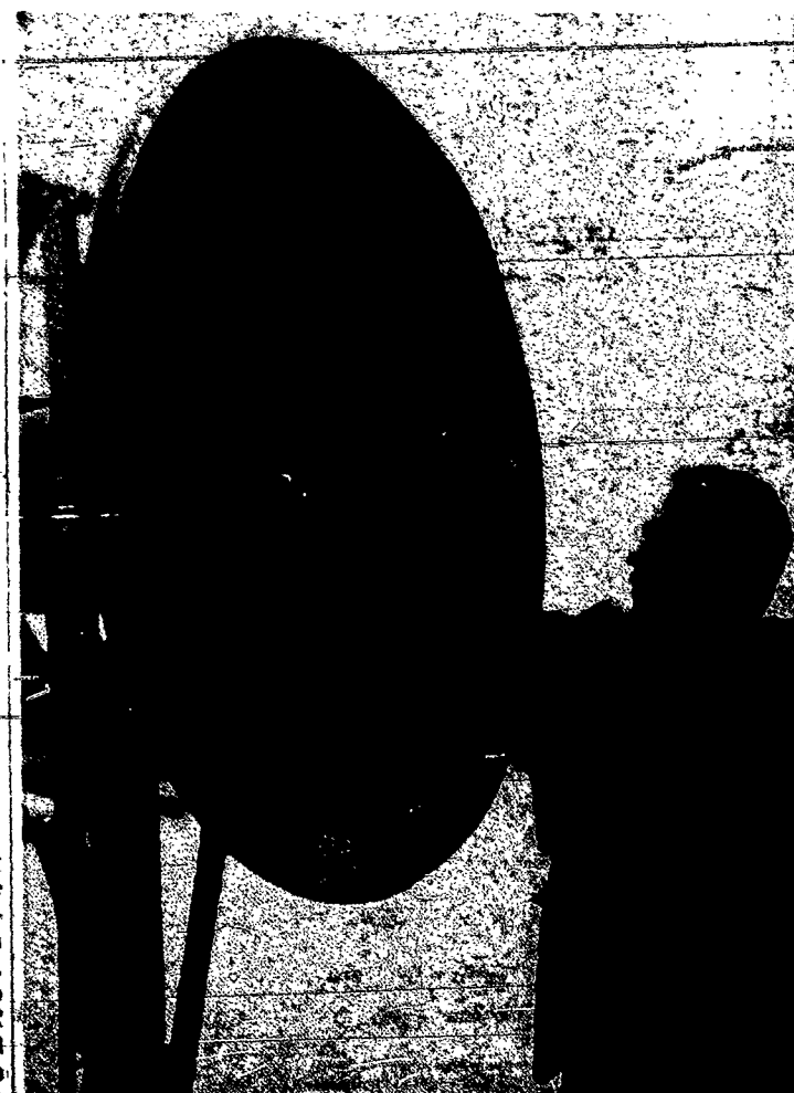
Elmer Grubb, WHAM-TV engineer, adjusts the parabolic reflecting dish on the roof of Rochester's Radio City which sends the video impulses from the studio cameras out to the transmitter on Pinnacle Hill for amplification and relay to receiving sets in the area. A portable version of this "dish" on top of the station's mobile-unit can send a signal to the transmitter from remote broadcast points outside the studio.
