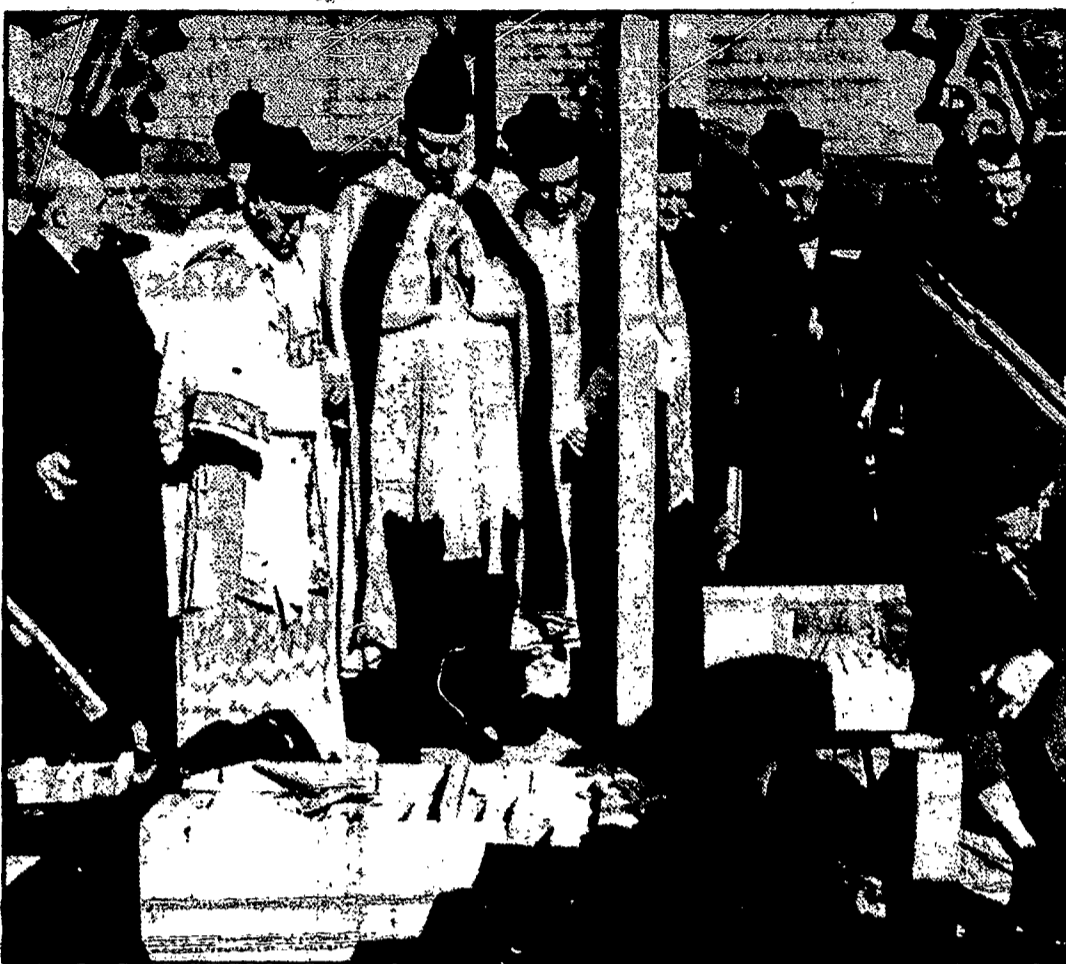
Marking the rebuilding of St. Anthony's school, Elmira, after the disastrous fire of Feb. 26, 1947, cornerstone is laid with impressive ceremony. Adolph Cirulli, trustee, stands ready with copper container in which historical documents were placed to be enclosed in cornerstone. Participating (from left) Rev. James C. Lane, Rev. William J. Naughton, Rev. Albert L. Simonetti, pastor of St. Anthony's; Monsignor William J. Brien, V.F., dean and officiating prelate; Rev. Thomas J. Toole; Monsignor Francis J. Lane, Rev. Theodore J. Winterroth and Rev. Leo E. Lynch.
