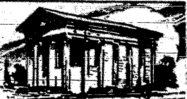
ST. MARY OF EGYPT CHURCH, ROME, was formerly A PAGAN TEMPLE. Church in 872 the space between the columns was walled up to increase the size.
