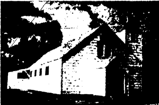
Rev. John F. Casey, S. S. E. is the building priest of the Fathers of St. Edmund in Alabama. Above he is seen trimming boards on a power saw. Below is Our Lady of Lourdes Chapel, Mobile, Ala., which he recently completed. Father Casey is now pastor of All Saints' Mission at Anniston Ala. where he is starting to build a convent for the sisters who are to arrive soon.
