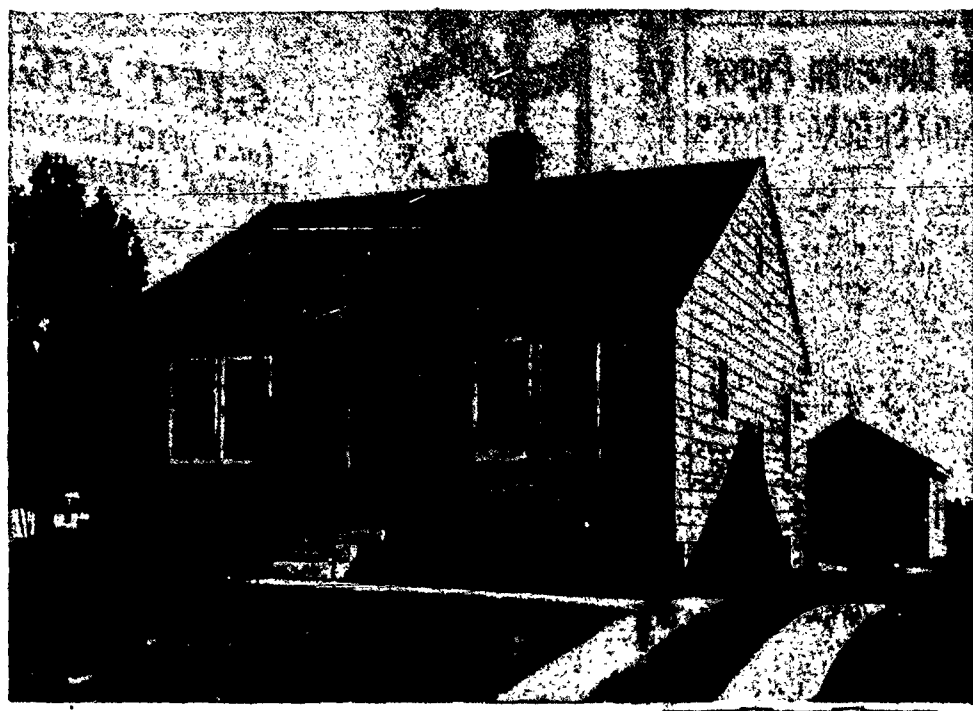
The bedrooms of this small home are well arranged and in good relation to the rest of the house. The bathroom opens on a common hallway, making passage through either bedroom unnecessary. The dining room in this compact living unit is advisable as both kitchen and living room would have suffered greatly from loss of space had a dining room been included. The Federal Housing Administration insured a mortgage of $4,500 on this property, the mortgage to be amortized over a period of 24 years by monthly payments of $27.80. These payments do not include taxes and hazard insurance.
