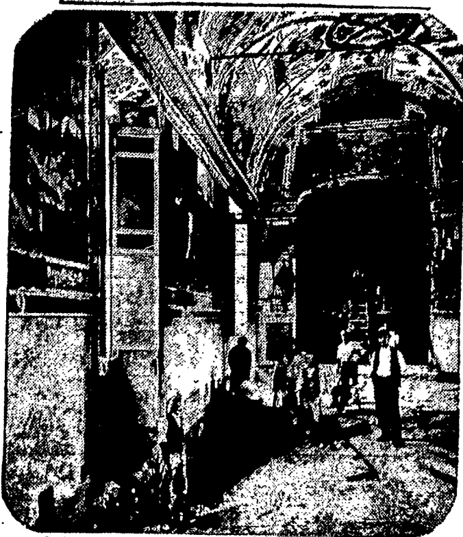
Workmen are shown here completing the reconstruction and strengthening of the Sixtine Palace of the Vatican Library which was damaged by the collapse of the roof just a year ago. A Requiem Mass for five victims of the disaster was recently offered in the Church of Sant' Anna in the Vatican, and was attended by all those connected with the library. (Aeme photo)
