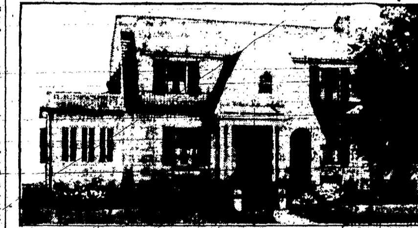
Six good large rooms and a large sun parlor are shown on the floor plan of this frame home. The center entrance leading into the hall and a living room that extends across the side and connected with the sun parlor are features. The house is 24 feet wide and 30 feet long.
