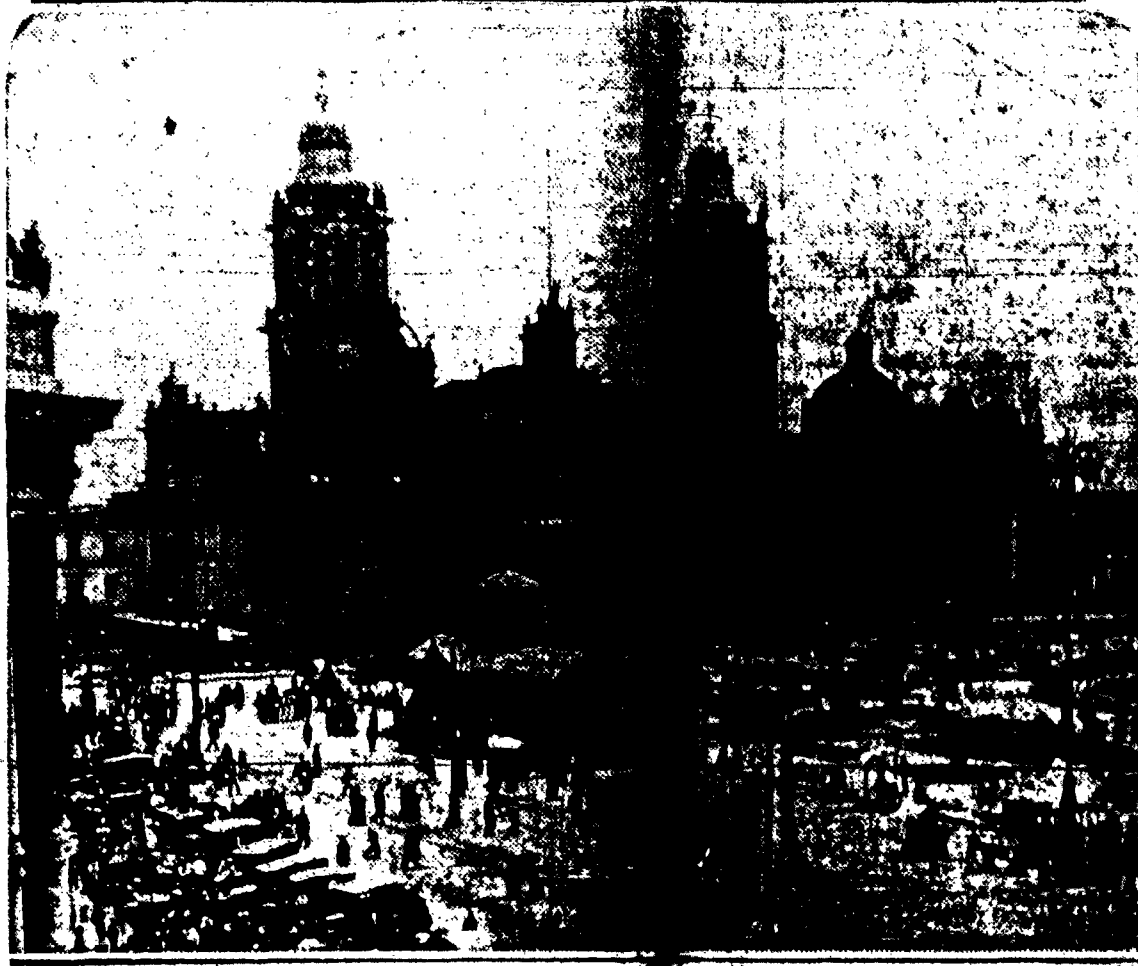
Engineers of the Mexican Government are endeavoring to determine the condition of the foundation of Mexico City's great Cathedral, the largest in North America. Earthquakes have damaged this Cathedral in the past. There is a possibility that religious services will be resumed in the Cathedral in the near future.
