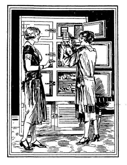
Let us install SERV-EL Automatic Refrigeration in your own ice box. SERV-EL cooling tank can be installed in the ice compartment with mechanism in basement or other convenient place and it will keep your ice box colder than is possible with ice.
