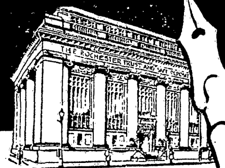
Main Street West & Exchange
