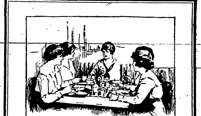
A Corner in a Dining-room in a Telephone Central Office
