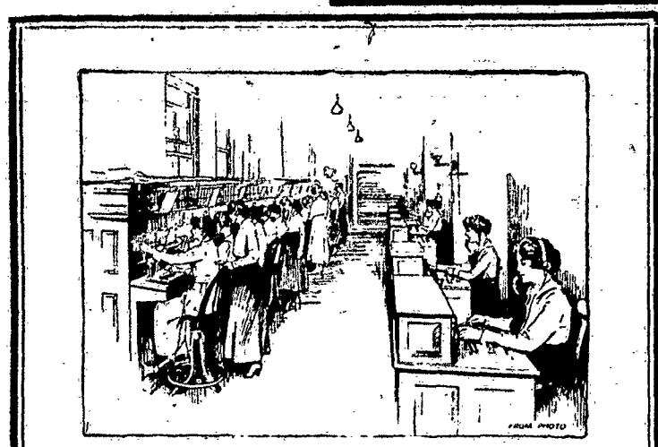
A Practice Switchboard in the Operator Training Department.
