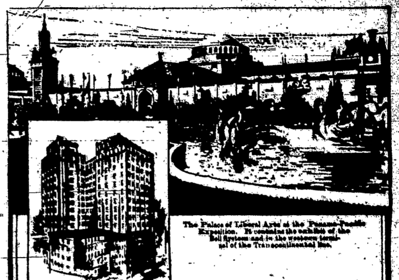
The Telephone building in New York is the center terminal of the Transcontinental line.
